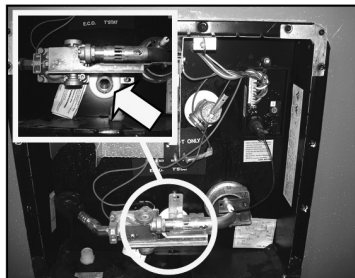
Water Heater Drain Plug Location
